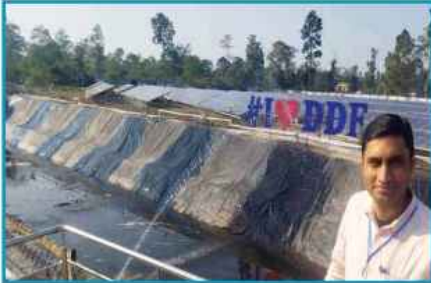
Rainwater Collection pond
