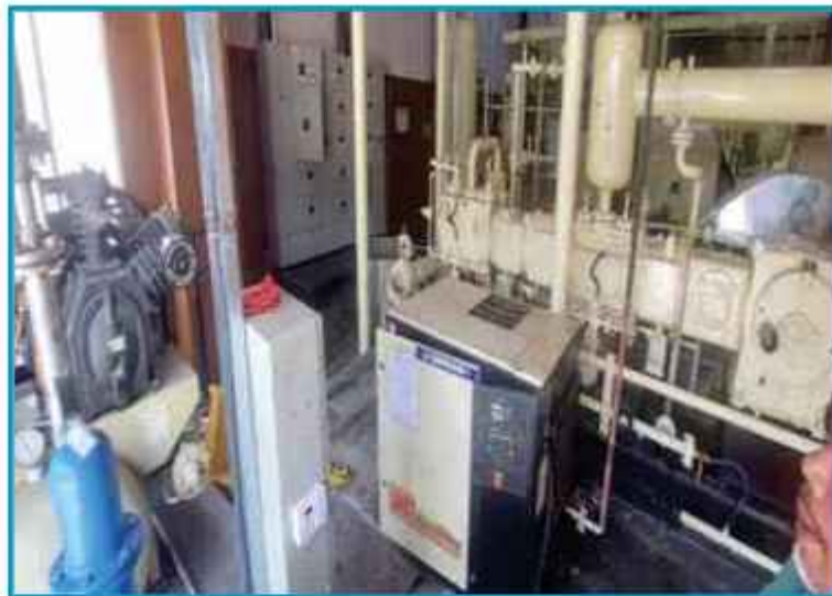
Measurement and Observation during Energy Audit
