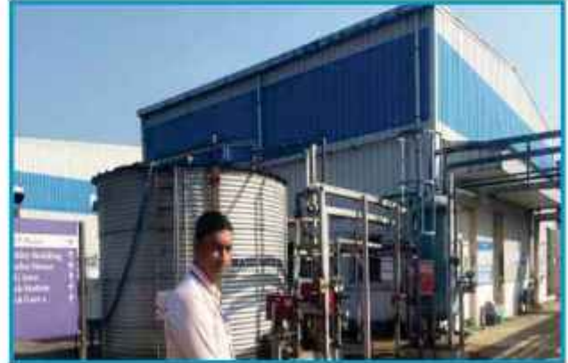
ETP Plant Area
