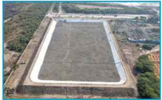
Newly constructed Secured Landfill Facility as per NPC Design
