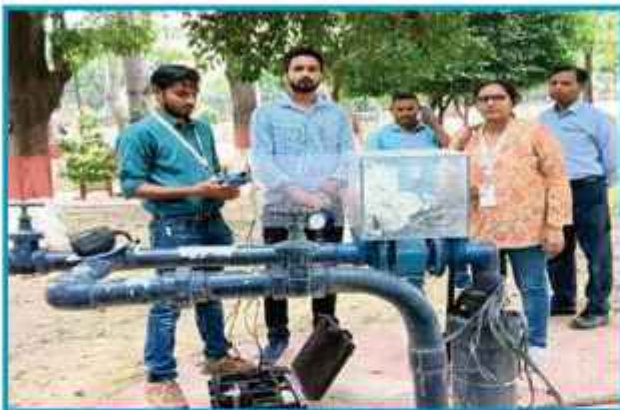
Ms. Preeti Gangwar, DD, NPC Kanpur during Water audit study as per Building Code at Office Building and premises of M/s Reserve Bank of India, Lucknow
