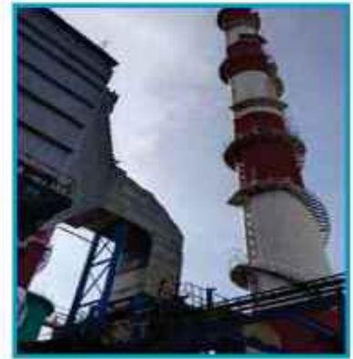
Stack attached to ESP
